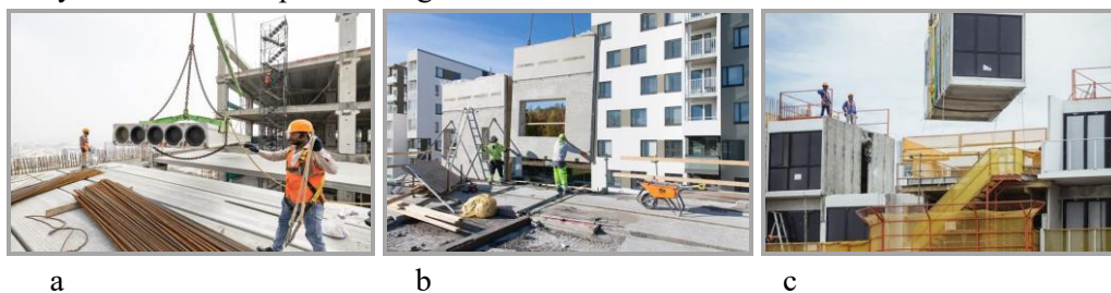
Fig 3. Precast concrete systems (a) Frame system, (b) Panel system, (c) Cell system [10] [11]
