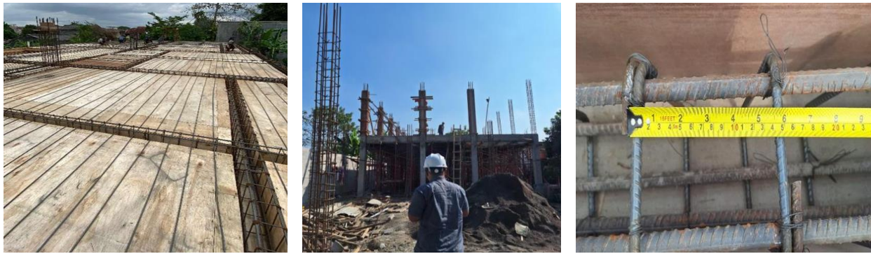
Fig 3. Student Involvement in Reinforcement Inspection Prior to Concreting Source: Internship field documentation (2025).
