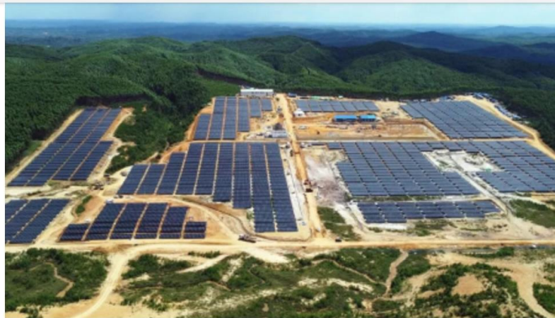
Fig 11. IKN Solar Power Plant (Sourcer: https://ikn.go.id/ ).
